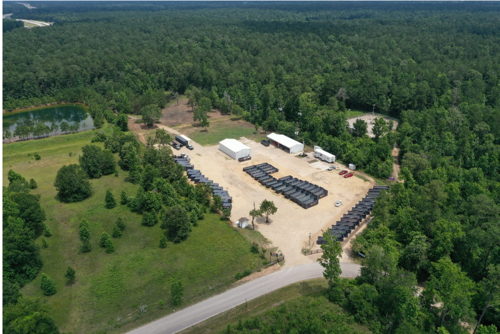
Photo 01. Aerial image of subject site looking northwest.
